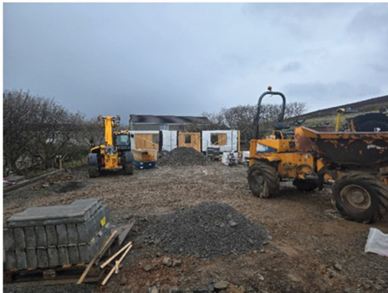
Johnstons Road progress
